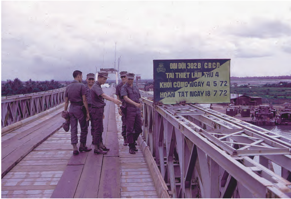
Colonel Nghia inspects repaired bridge at Go Dau Ha, which was completed by the 302d Engineer Battalion on 18 July after being destroyed during the Easter offensive.
